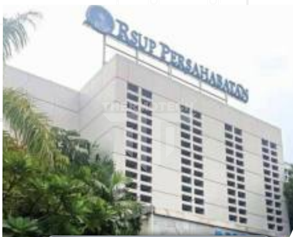
PROJECT NAME : RSUP PERSAHABATAN APPLICATION PRODUCTS : DUCT INSULATION LOCATION : RAWAMANGUN
